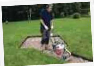
Once the sub-base is smooth, flat and to the appropriate level, check the drainage slope with a straight edge and spirit level.
