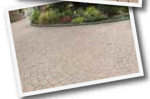
This illustrates how colours can differ in the photos due to climatic conditions, but also how different manufacturing processes involved – for instance, Alpha Antique which is tumbled to give an aged appearance and Classico which is not – can alter the appearance of colour.
