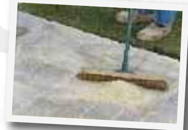
Subsequently top the sand and re-compact to ensure that no joints are left unfilled.
