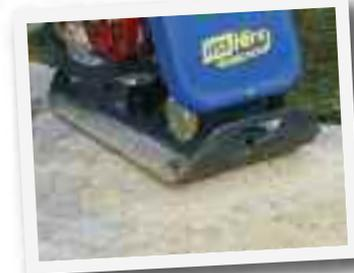
**Hints & Tips:** Always keep a bag of kiln dried sand around after you've finished your job, as sand will come out of the joints in the initial life of the area. Regularly top up until it settles in the joints.
