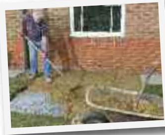
A further 20mm layer of sharp sand then needs to be raked on top and using the screeding rails and string line, levelled to the correct falls.
