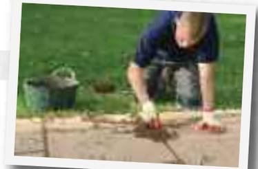
Firm it into the joints using the trowel and finish with the pointing iron, compacting the mix into the gaps and producing neat grooves.
