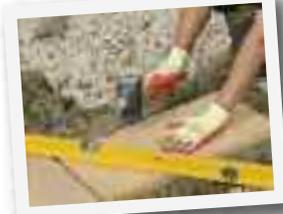
Line up the paving flag with the string lines and gently tap it into the mortar using the rubber mallet.
