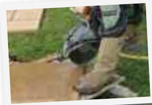
Mark the paving flag surface with the intended cutting line for guidance. Place the paving flag on a platform and carefully saw using a diamond disc cutter.
