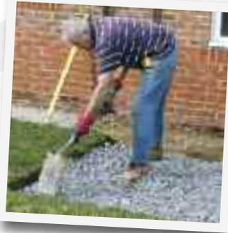
Using the cement mixer, mix 1 part cement and 6 parts ballast to create a concrete foundation for the edge restraint that is 100mm thick. Ensure that the edge restraint unit that is to be placed on the foundation will sit at the required finished level using the string line and spirit level.
