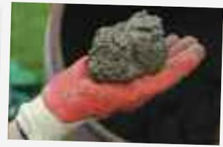
Starting in the corner, trowel a bed of mortar to cover the area intended for the first paving flag. The depth of the mortar bed should be approximately 35-40mm. Level off but ensure the mortar is not compact as you want the flag to sit within the mix about 10-15mm deep.
