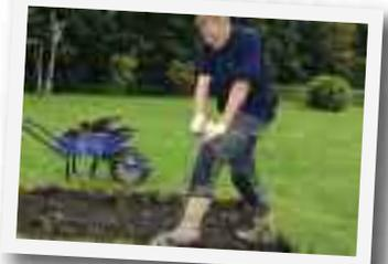
If you find soft spots in the soil, further excavation may be required. These spots can then be filled and consolidated with sub-base material.
