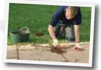
Firm it into the joints using the trowel and finish with the pointing iron, compacting the mix into the gaps and producing neat grooves.
