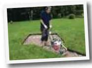
Once the sub-base is smooth, flat and to the appropriate level, check the drainage slope with a straight edge and spirit level.
