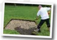
Once the area is covered, check the depth using a spirit level, pegs and string line.
