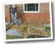
A further 20mm layer of sharp sand then needs to be raked on top and using the screeding rails and string line, levelled to the correct falls.
