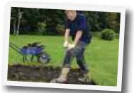
If you find soft spots in the soil, further excavation may be required. These spots can then be filled and consolidated with sub-base material.
