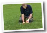
The excavated depth should be 150mm or 6 inches from the finished patio level. Measure the final depth of excavation using the pegs and strings.
